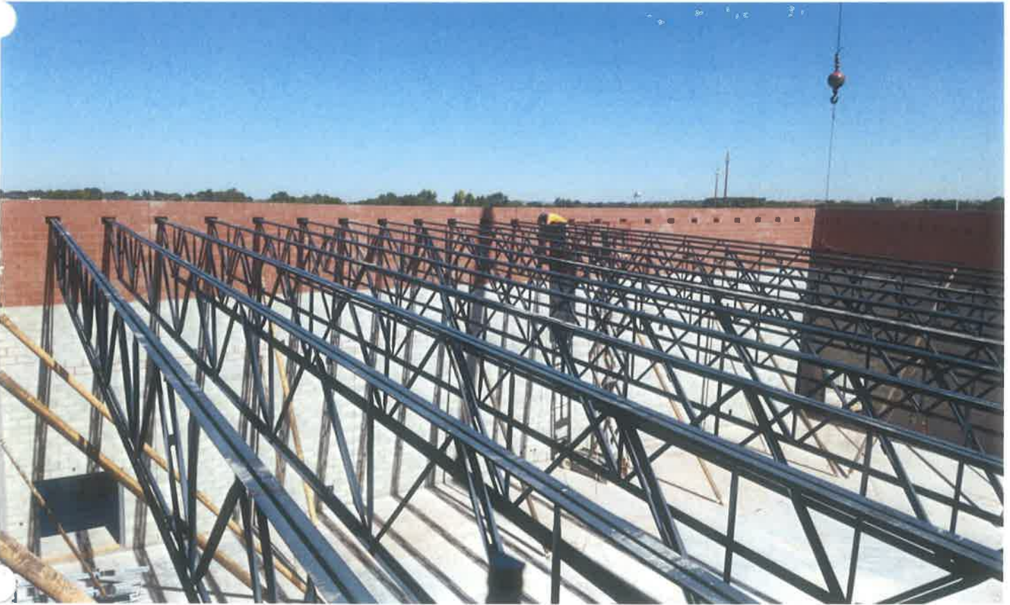
Gym Roof Joists(Above) & (Below)
