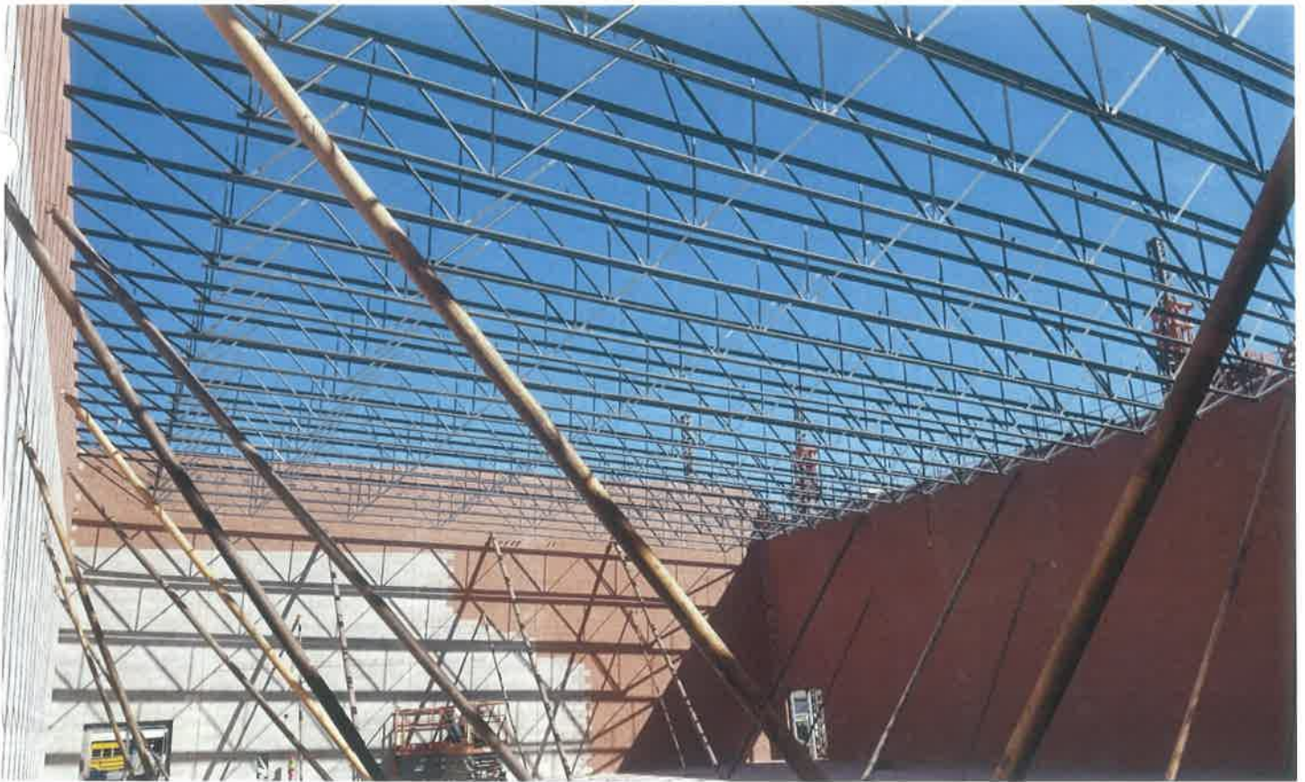
Gym Roof Joists(Above) & (Below)
