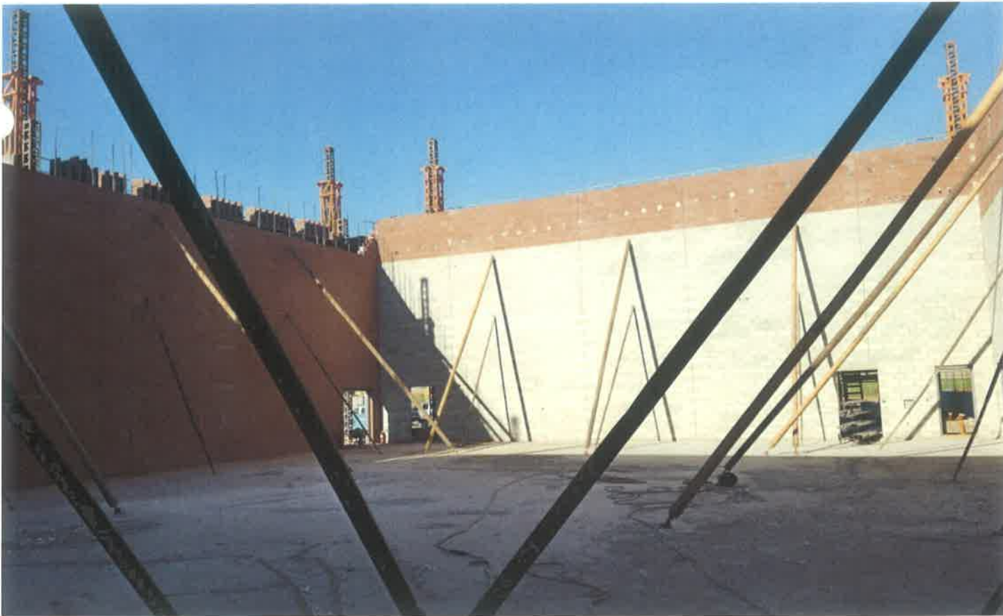
Gym Bracing from Floor (Above) & Gym from Scaffold (Below)
