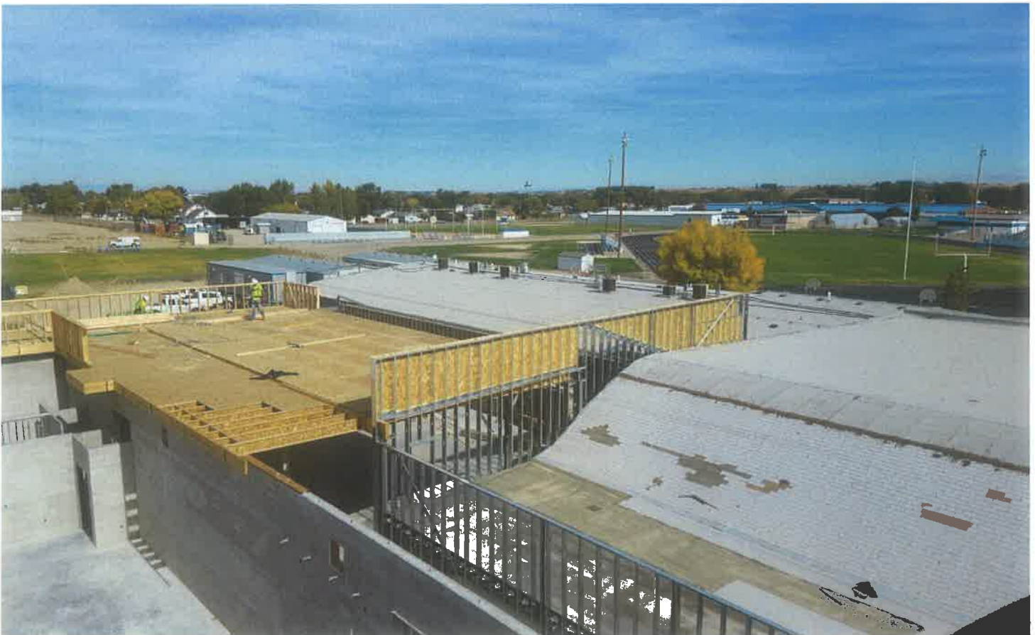
New Commons Parapet (Above) & Mechanical Well Above Art Rooms (Below)
