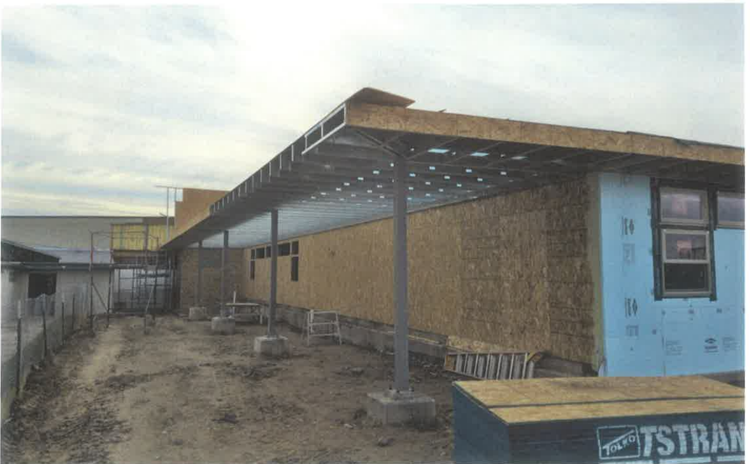
North Elevation Set-Up for Veneer (Above) & East Overhang (Below)
