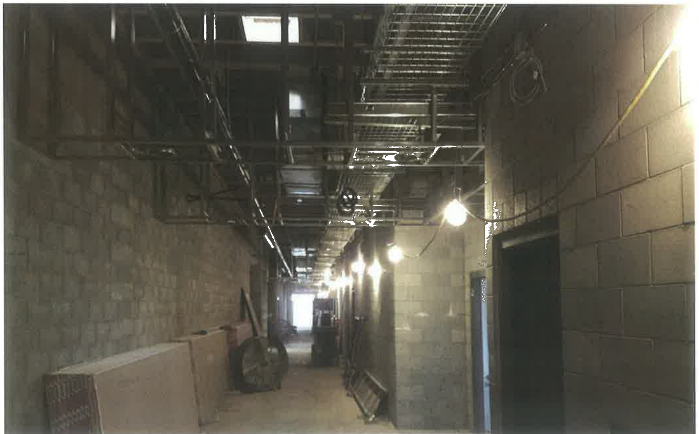
Hallway Rough-Ins (Above) & Hallway Alcove Framing (Below)
