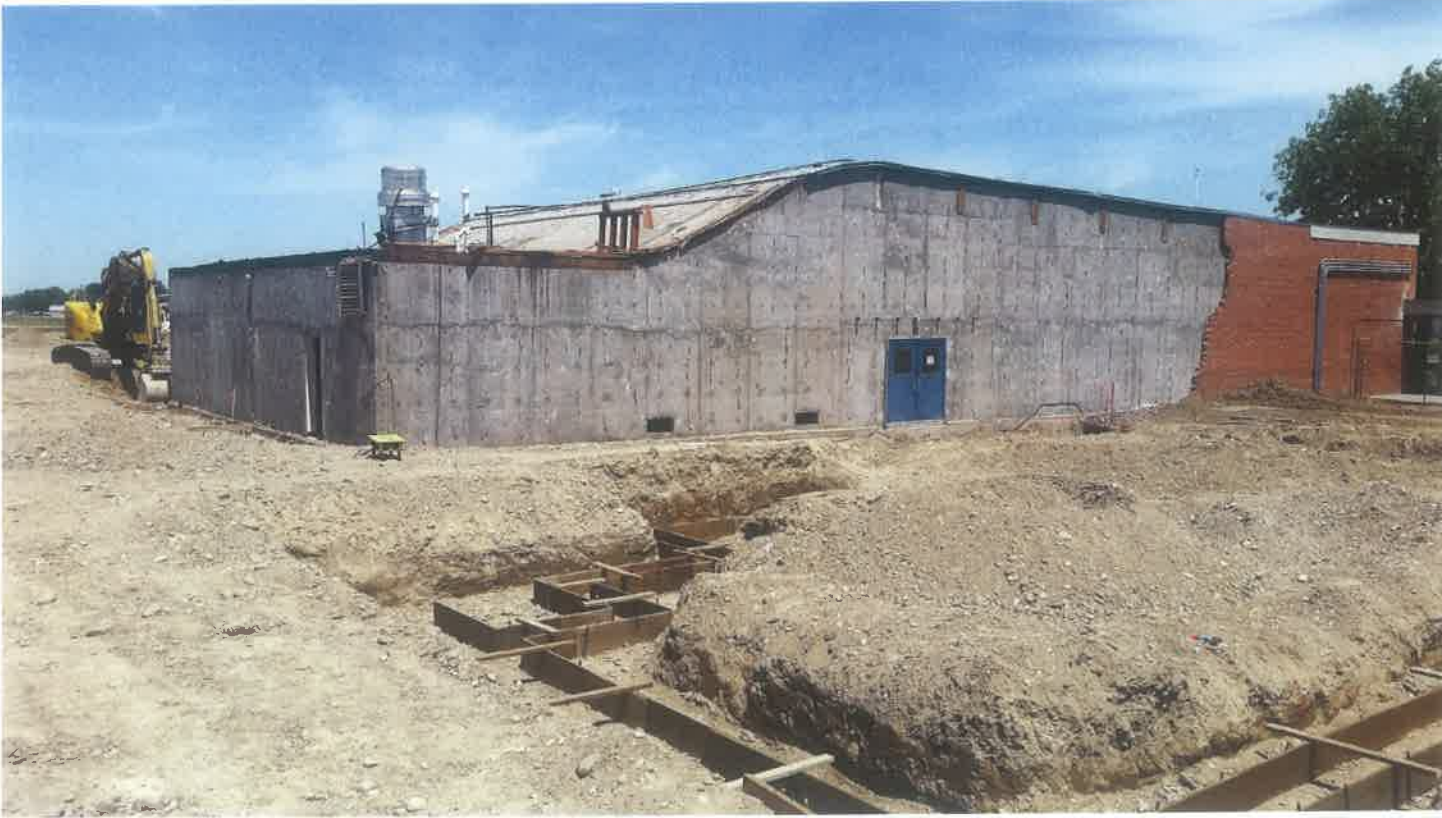
Footing Formwork (Above) & Commons / Footing Forms (Below)
