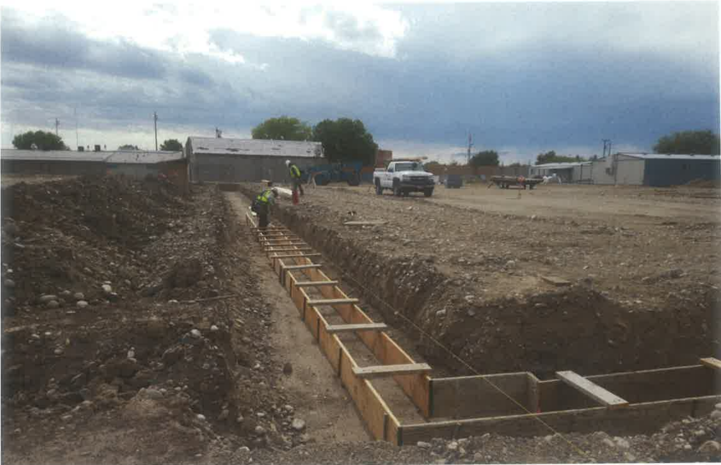
Footing Formwork (Above) & Commons / Footing Forms (Below)
