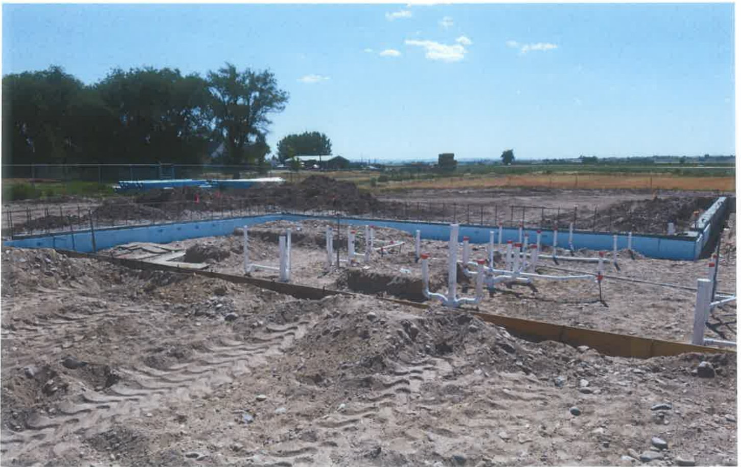
Locker Room Stub-ups (Above) & Footings (Below)
