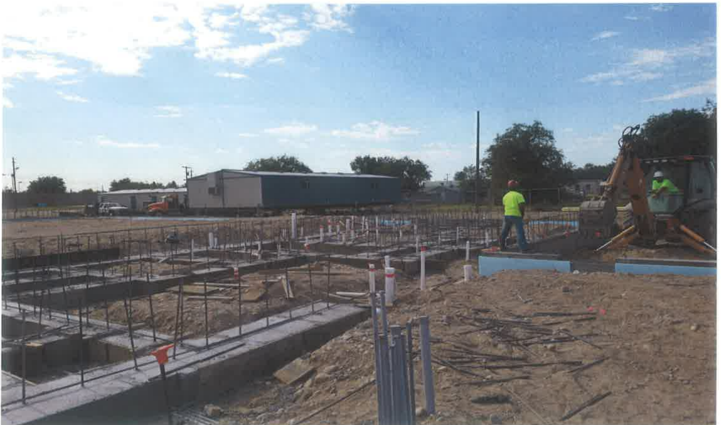
Locker Room Stub-ups (Above) & Footings (Below)
