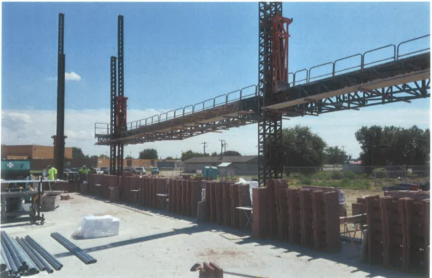
Gym Scaffold System (Above) & Scaffold, Staged Block (Below)
