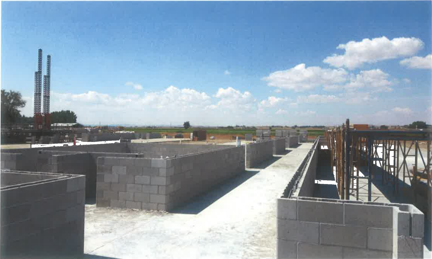
Red CMU and Mortar (Above) & CMU at Corridors (Below)
