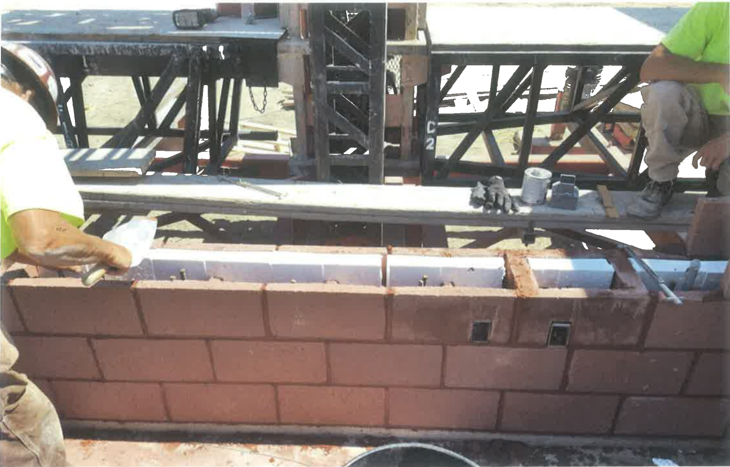
Red CMU and Mortar (Above) & CMU at Corridors (Below)
